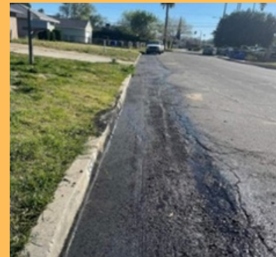
Hot Patch work at 35th and Conejo (Ward 4)
